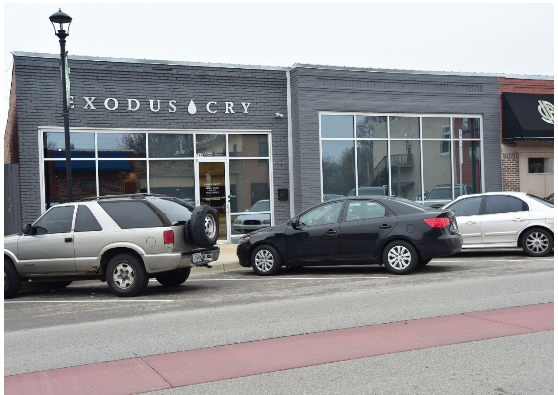
714 Main Street, Official Survey Photograph, 2018
